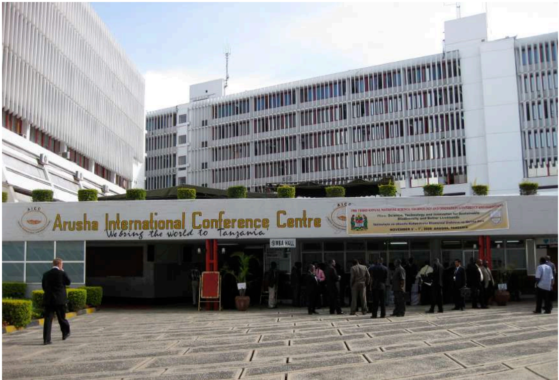
Figure 1.4: The Arusha International Conference Centre :Venue for peace talks to end the war.
